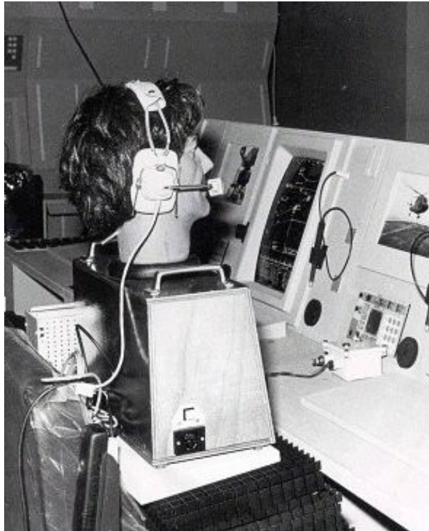
Figure 19. Artificial mouth used for the assessment of microphones.
